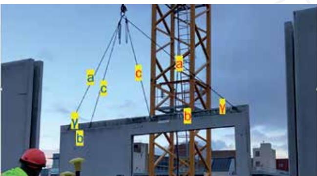
Figure 7. Lifting Configuration with the Cosine Rule Built-In
