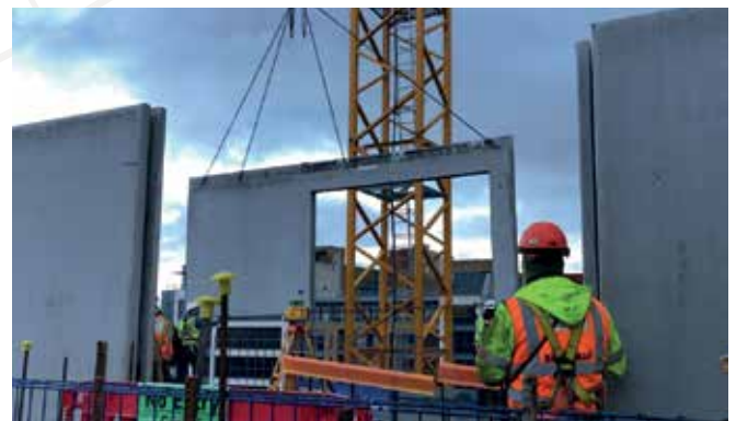
Figure 1. The 4 Lifting Eye Unbalanced Panel During Lifting
