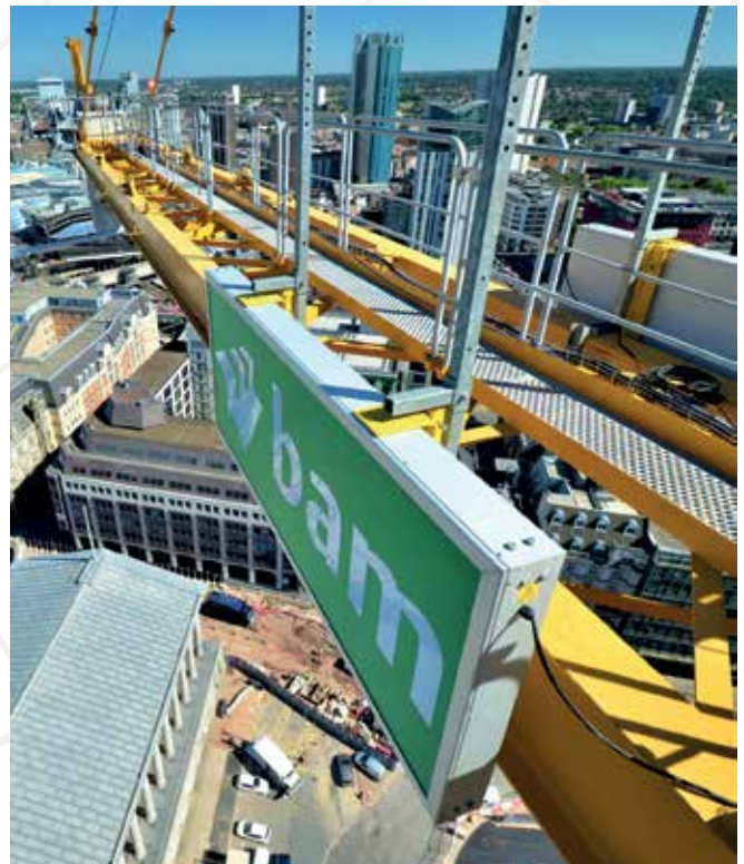
Figure 2: BAM construction site
