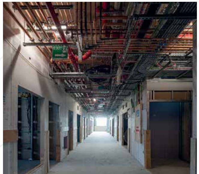
Figure 2: Construction Site that used the HIVE
