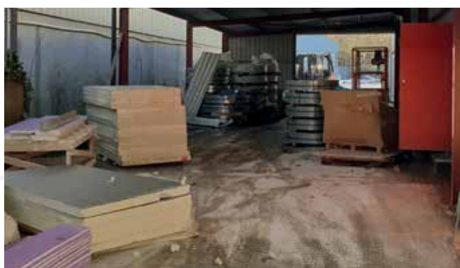
Figure 6: Before: External space inefficiently used for miscellaneous storage of spares and raw materials.
