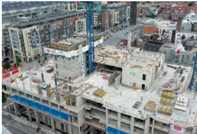
Figure 5. Actual View of Slab Showing the Locations of the Placing Booms
