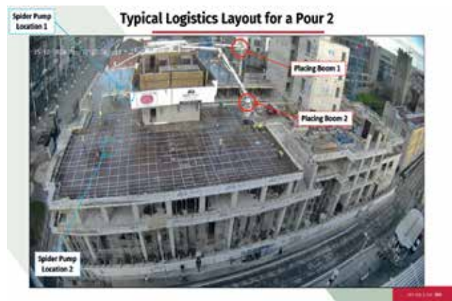
Figure 6. Placing Boom Locations
