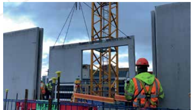
Figure 1. The 4 Lifting Eye Unbalanced Panel During Lifting
