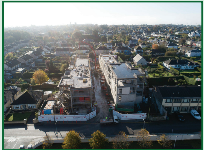
Figure 1. Drone Footage of Top-Out Pour on Reinforced Concrete Frame
