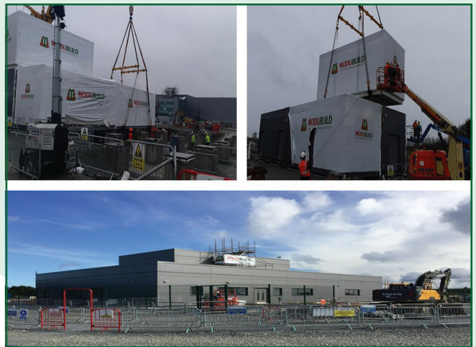
Figure 3. On-Site Module Installation, & Assembled Building
