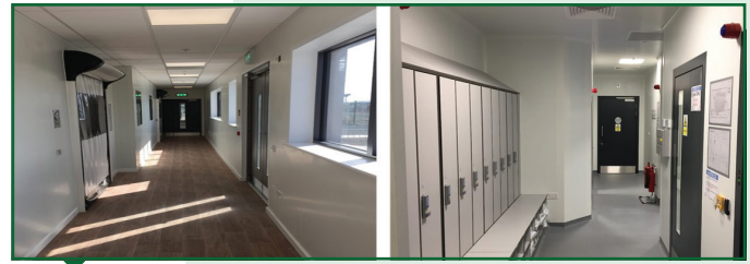
Figure 4. Module Internal Finishes – completed off-site
