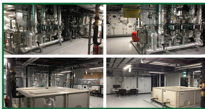
Figure 5. Plant Room & FAT Testing Station completed off-site
