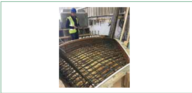
Figure 3. Timber Mould with Rebar Cage In-Situ Before Concrete Pour.
