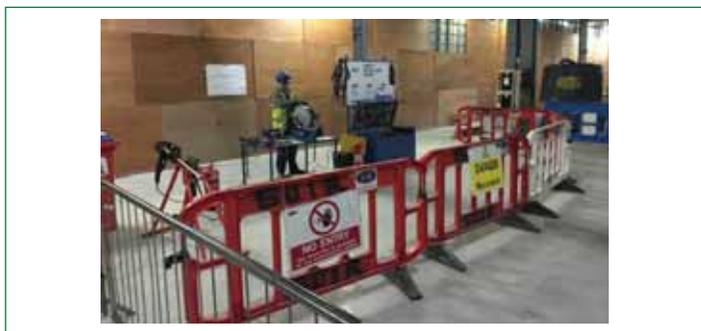
Figure 1. Material job-box and workbench set up close to work area.
